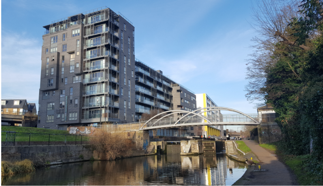
Photograph of the development opposite the site.
